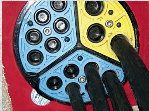
HSI 150 - SEGMENTO - with integrated torque control system and bling plugs
