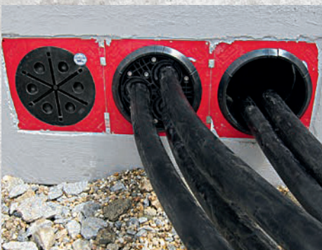
HSI 150 - wall insert with SEGMENTO - sealing of control lines in a substation
